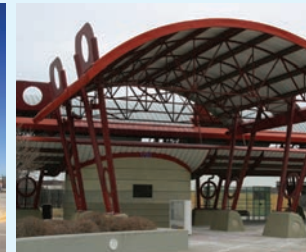
Northwest Transportation Center
